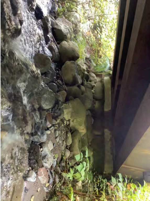
Right Bank Abutment when facing downstream
