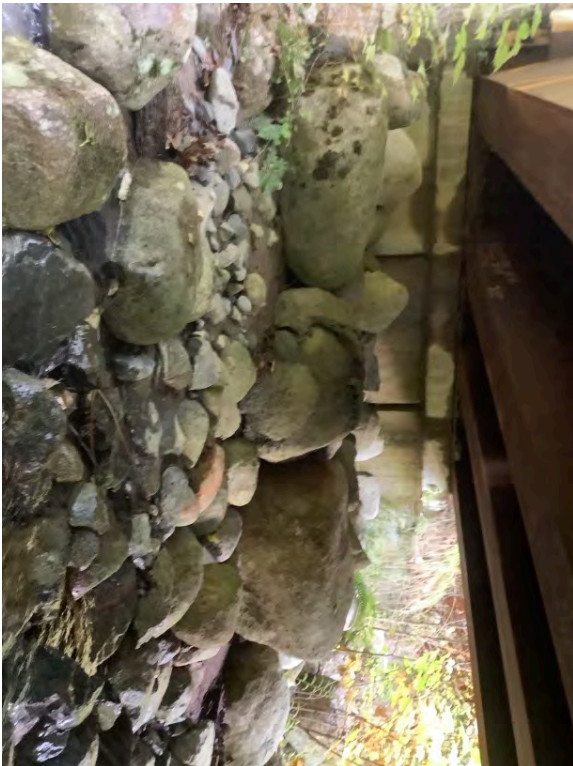
Left Bank Abutment when facing downstream
